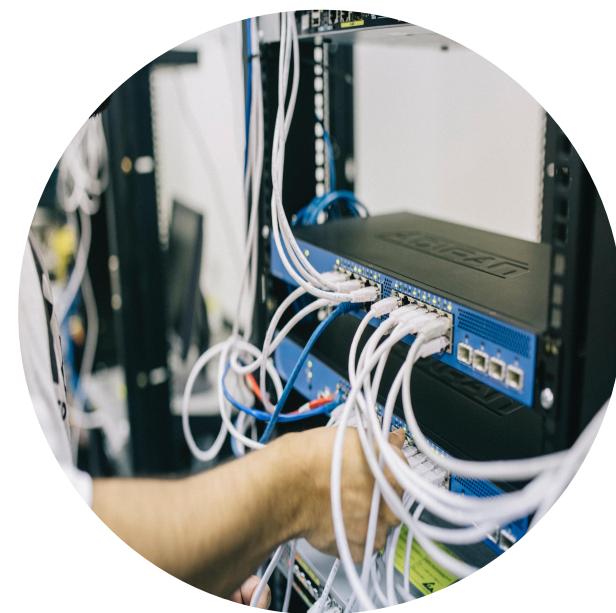
安装调试 Installation and debugging
